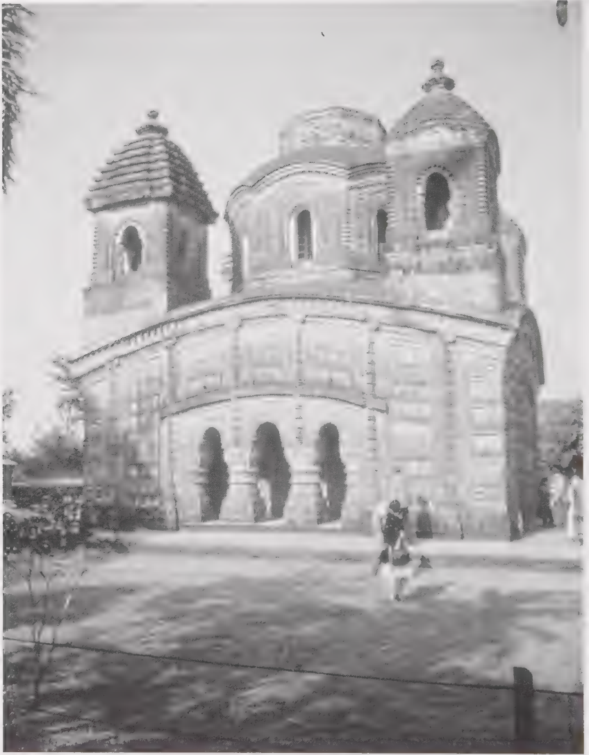
Figure 7.13 The double story Shyam Ray temple, dated 1643, is especially designed to facilitate a new form of devotion in Bengal for the deity Krishna and his consort Radha.
