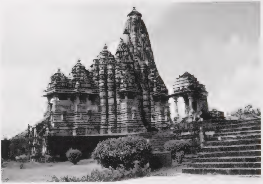
Figure 1.2 The Kandariya Mahadeva temple, Khajuraho, dating to the early eleventh century, has a superstructure composed of clustered spires typical of north Indian temples.
